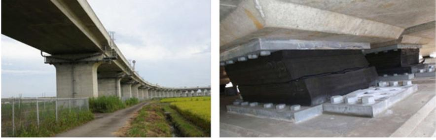
**Fig. 5** Great East Japan Earthquake in 2011: bridge rubber bearings on the left and the horizontal crack is observed on the right [33]
